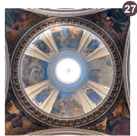
Chapel of the Blessed Sacrament, trapezoidal in shape, frescoed and surmounted by a small dome
